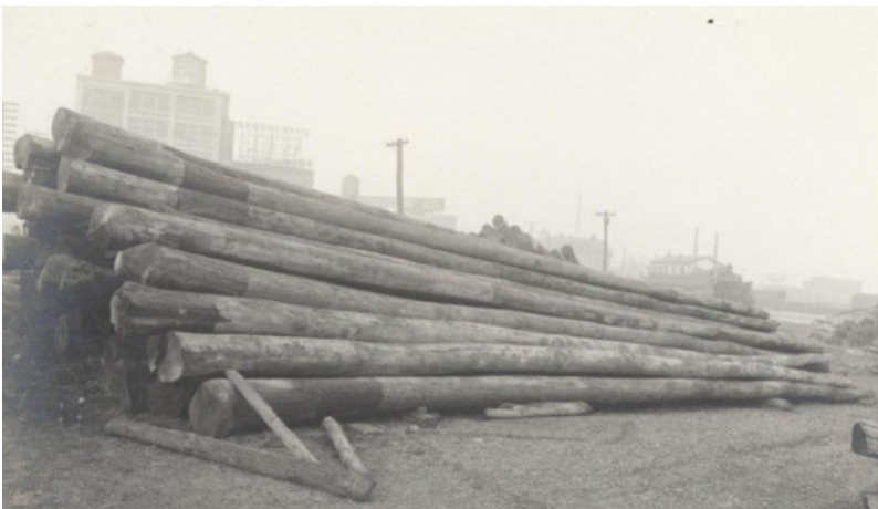
36: Telephone and telegraph poles made from blighted chestnut trees. (above)
