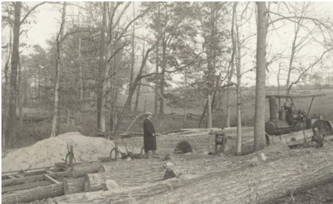
40: Portable sawmill sawing blighted chestnut trees into timbers for barn framing –Oxford, Chester Co. Pa. ( above )
