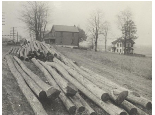
36: Telephone and telegraph poles made from blighted chestnut trees. (above)
