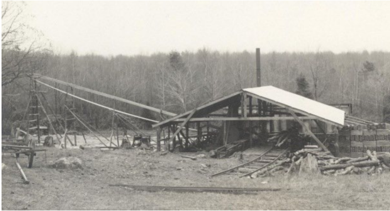
37: Stave mill and staves from blighted chestnut wood on the Estate of Col. H.C. Trexler, Allentown, Pa. [Photographs taken by William Currie. In the Report of the Pennsylvania Tree Blight Commission, July 1 to December 31, 1912 , the image on the left is captioned, "General view of portable stave mill operating in blighted chestnut. This kind of mill can utilize chestnut unfit for saw logs or shingles." The image on the right is identified as "Staves made from blighted chestnut, bundled, ready for shipping." c1912] (above)
