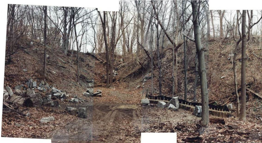
Hay bales and silt fencing near a gully on the South Street Tract. ca. April 1999 (Series IV, folder 8)
