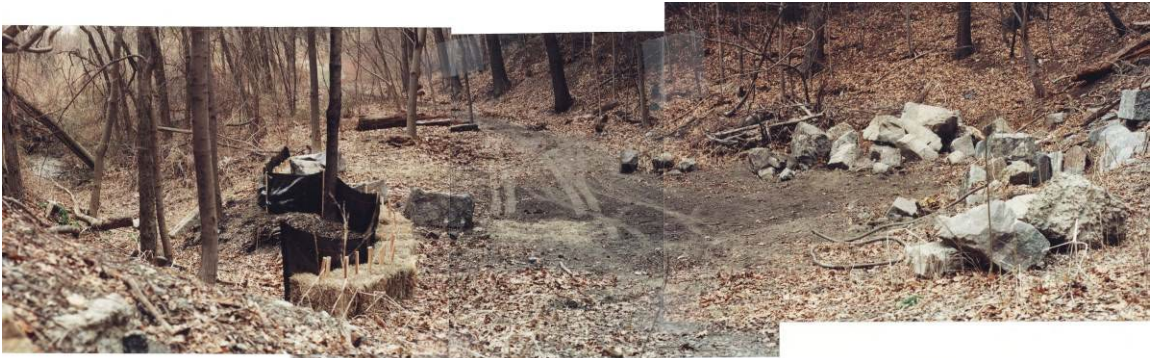
Hay bales and silt fences in a gully near an MWRA manhole. April 2, 1999 (Series IV, folder 8)
